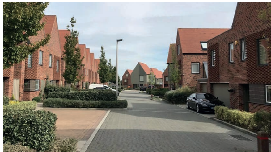
Precedent Image: Shared surface street. Horsted Park, Chatham - Proctor and Matthews Architects
