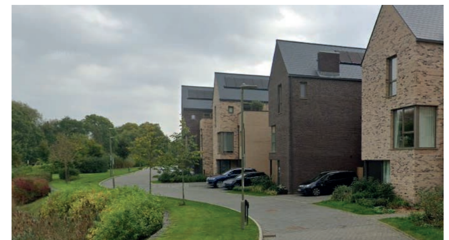
Precedent Image: Block paved street facing landscaped edge. Barton Park, Oxford
