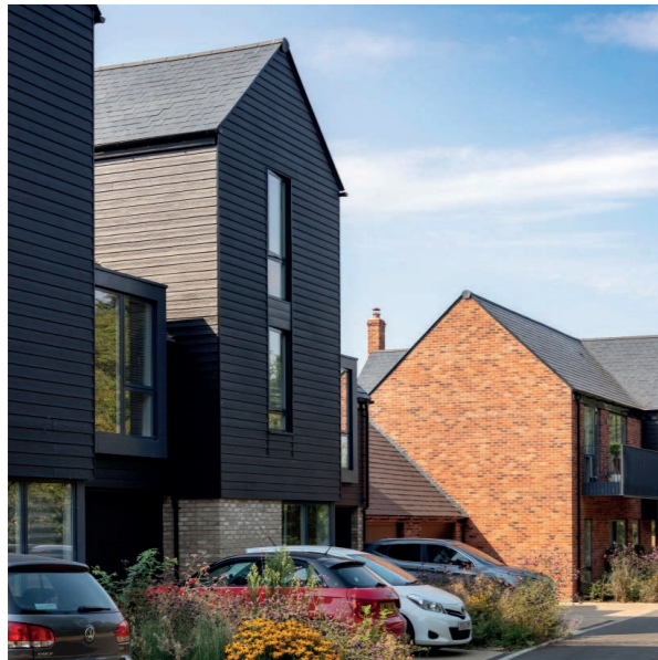
Precedent Image: Example of parking to the front of dwelling with planting between
