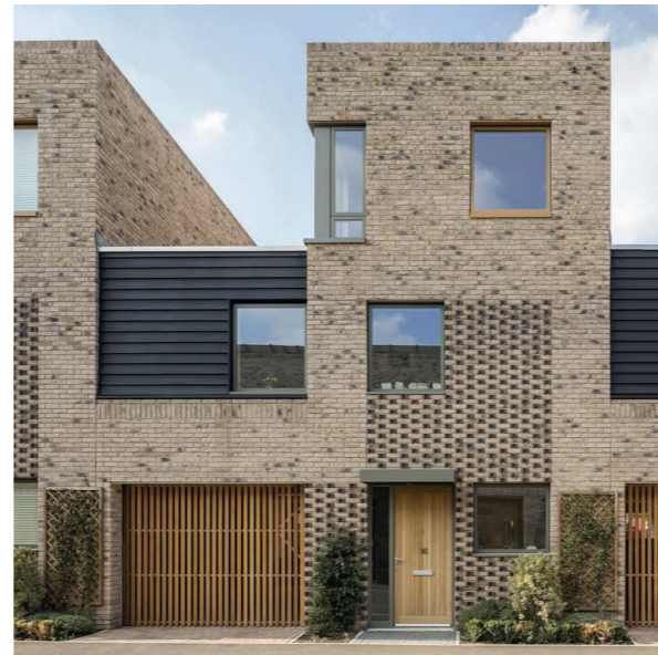
Precedent Image: Example of a high quality, well detailed integral garage
